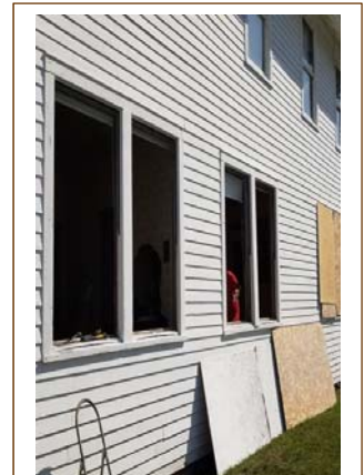
Funding window repairs, conference room enhancements and so much more!
